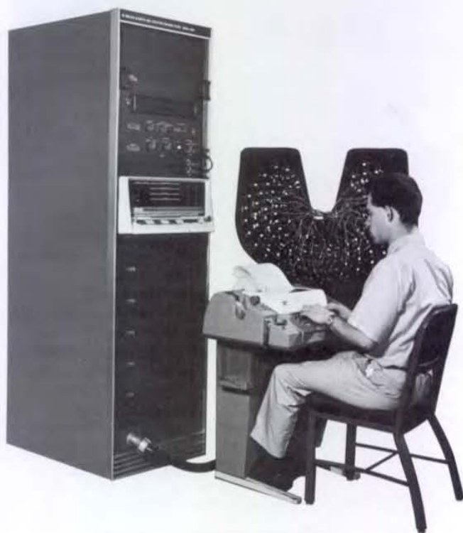
Figure 2. Automatic test assembly for communication cable inspection.
